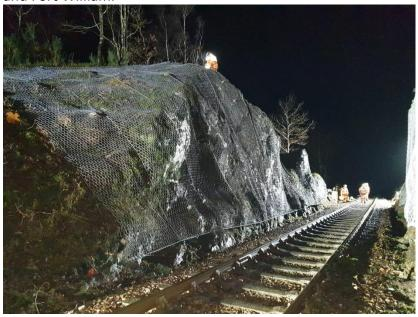
The work will protect 14 rock cuttings over a two and a half mile stretch of single-track railway between Locheilside and Lochailort encompassing both Glenfinnan station and viaduct. It will improve the resilience and reliability of this line for passenger services.
